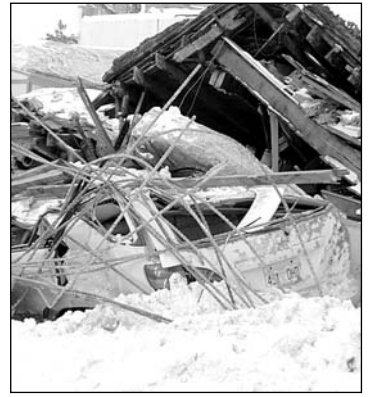
A collapsed building rests on a vehicle after a snow storm on Monday, in Trinidad, Colo.
